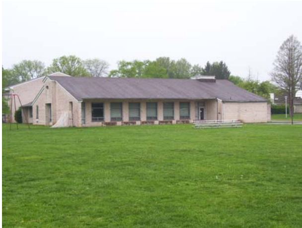
Typical lawn area in the central portion of the property.
